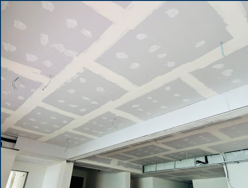
A 0508 – False Ceiling works in progress
