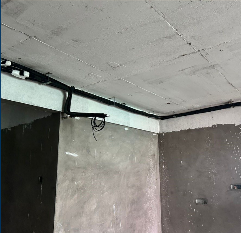
A 0805 – AC Copper piping works in progress
