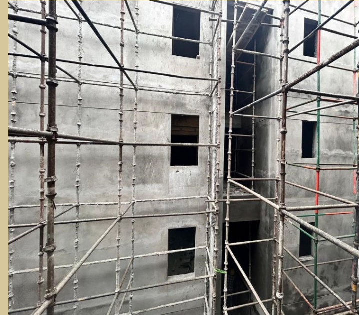
Atrium external plastering works in progress
