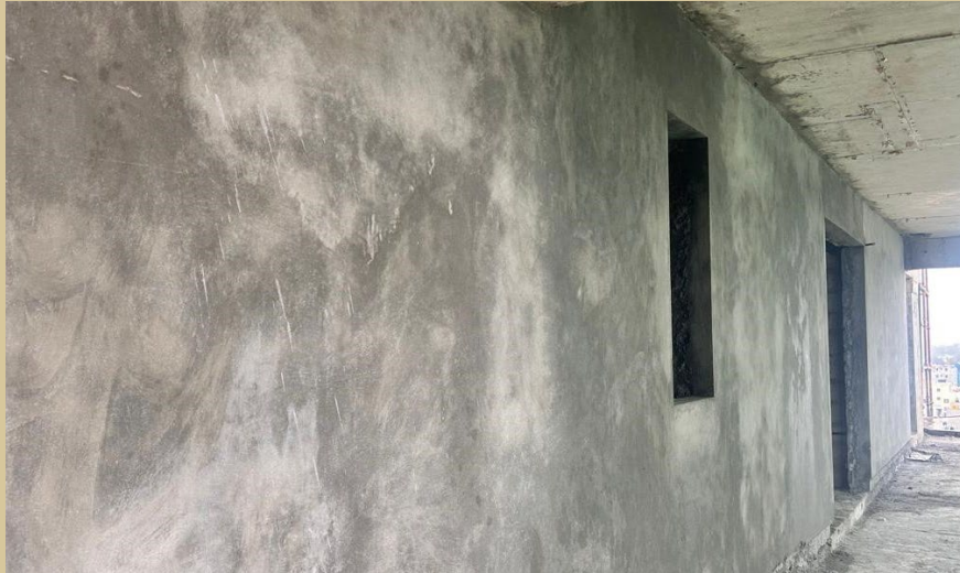
14 th Level External Plastering works in progress
