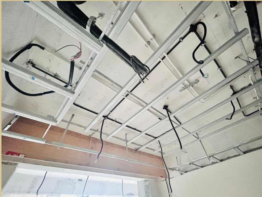
A 0510 – False Ceiling works in progress
