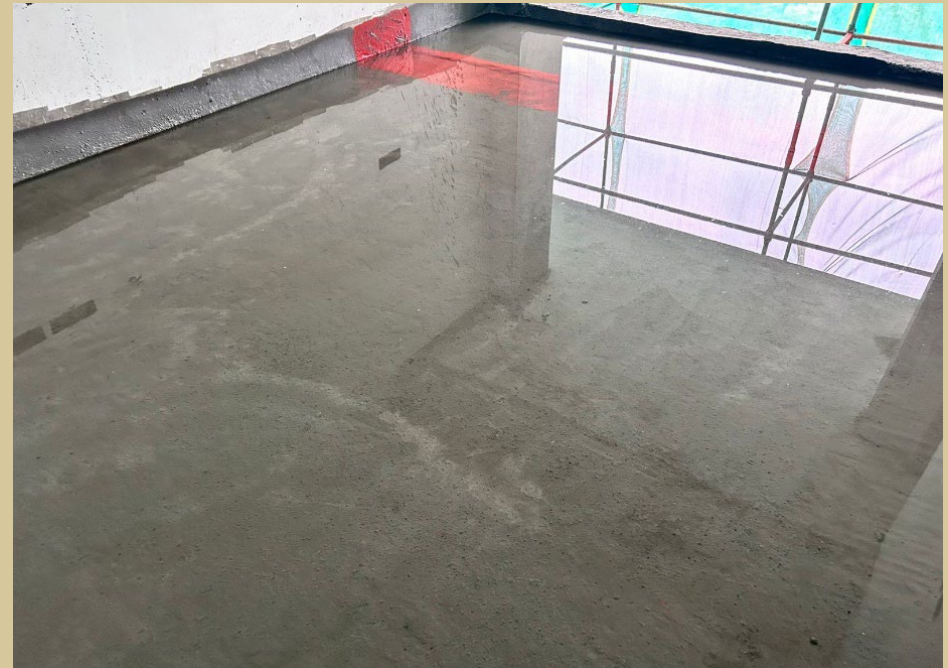
A 0609 – Waterproofing check in progress
