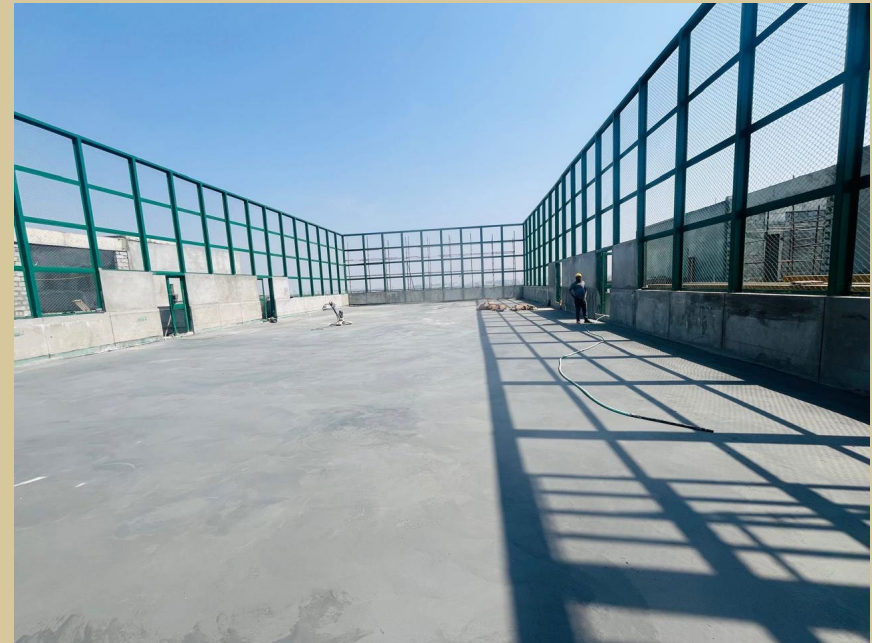
Tennis Court: Screed Concrete Completed
