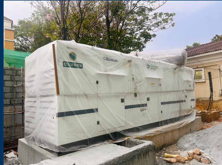
Generator Installation in Progress
