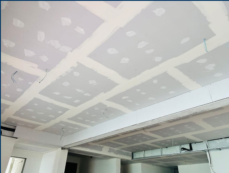
A 0508 – False Ceiling works in progress
